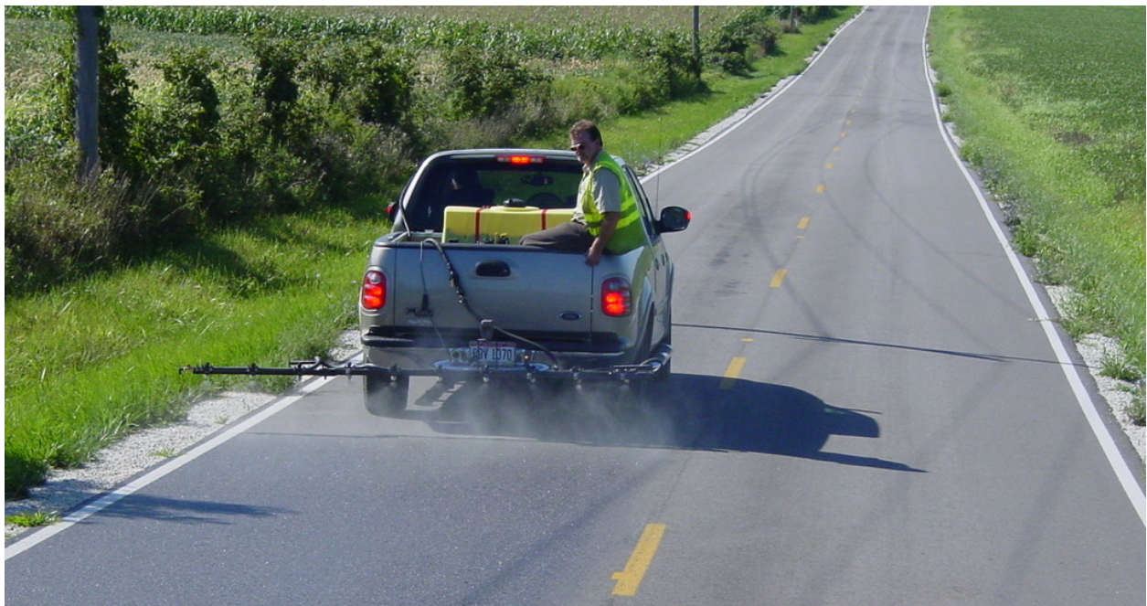
Figure 1: RePLAY being applied to a road surface
